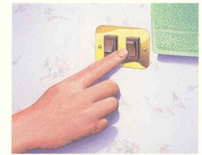
A water pump switch conveniently located in the bathroom is a good example of small things that make a big difference.
