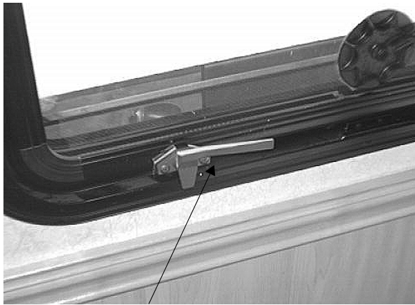
Lift latch handles upward to open. Escape Window
