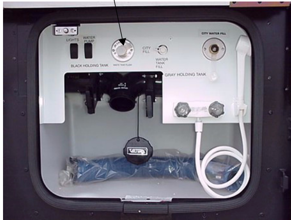
Water Tank Flush Inlet
