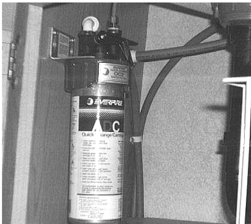
Water Filter Assembly - Below Galley Sink
