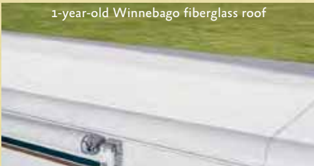
1-year-old Winnebago fiberglass roof
